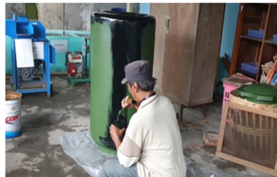
FIGURE 6. Materials The process of painting each part of the WWTP
