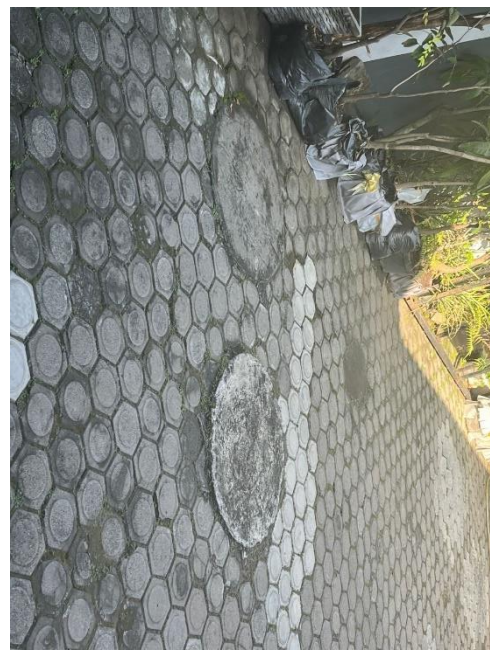
Pengecekan septic tank rumah penderita
